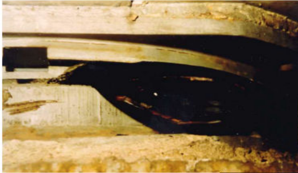
Failure of Elastomeric Pad Internal Seal
