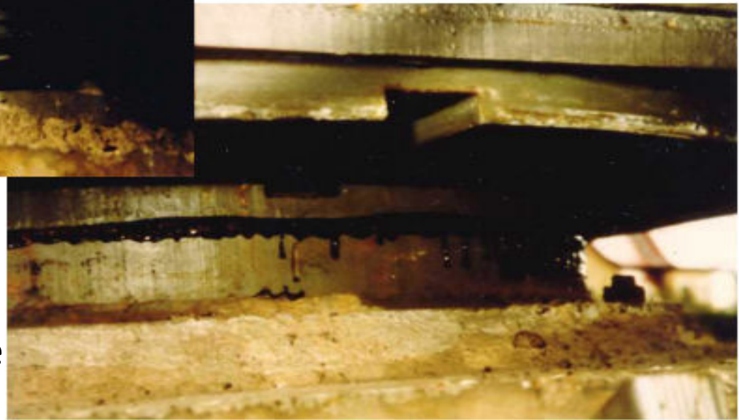
Failure of Elastomeric Pad Internal Seal
